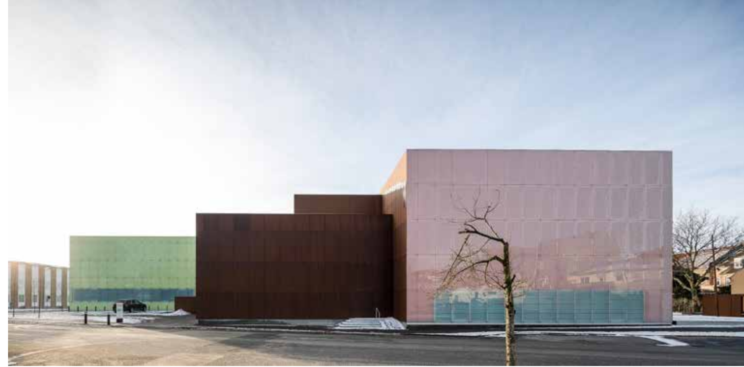
Frosted glass is paired with weathering steel in Schmidt Hammer Lassen's Vendsyssel Theatre in Hjørring.
