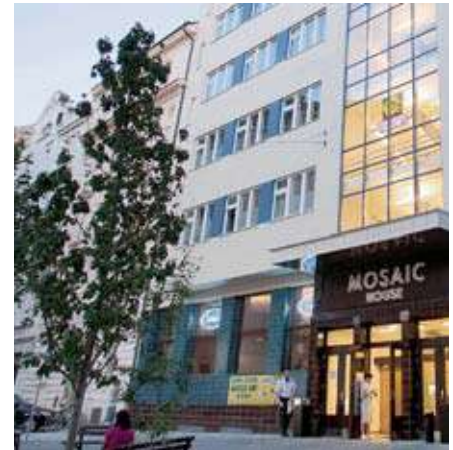
Hotels. Prague's Hotel Mosaic House is not only fitted out with various Hansgrohe products, but also runs the Pontos AquaCycle and Pontos HeatCycle.
