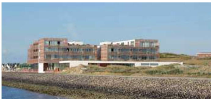
Hotel Budersand, Sylt. Hansgrohe products: Raindance Rainfall and Raindance S hand shower. Photo: jana-ebert.de
